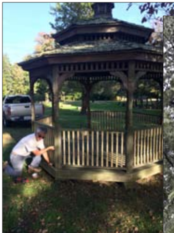
Arthur Damaskos repairs gazebo balusters at Dunseith Gardens
