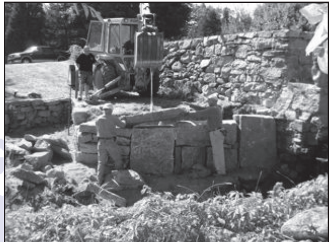
Tub Mill race repair – before and after
